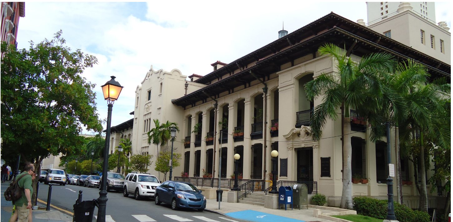
Jose V. Toledo Federal Building and United States Courthouse (Photo by Osvaldo Ocasio/Wikipedia)
